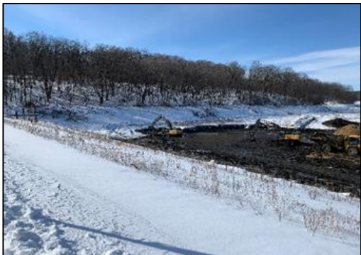
Dredging equipment at work at Lake Le-Aqua-Na State Recreation Area
