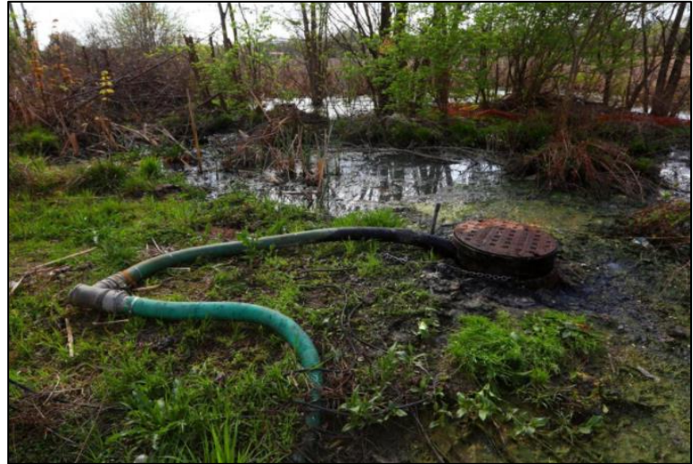
Cahokia Heights residential wastewater and sewage flooding
