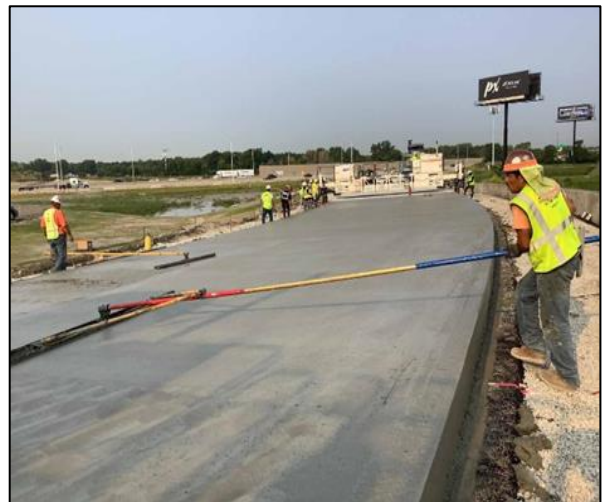
Work underway on I-490 Tollway near Des Plaines
