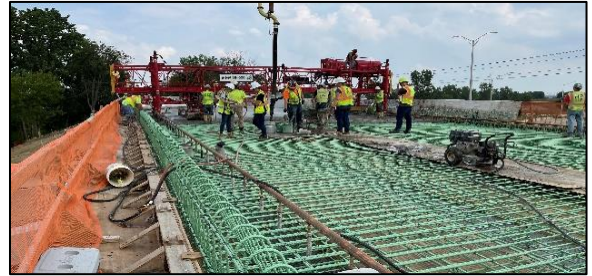
Deerpath Road Bridge over the Reagan Memorial Tollway (I-88) near Aurora
